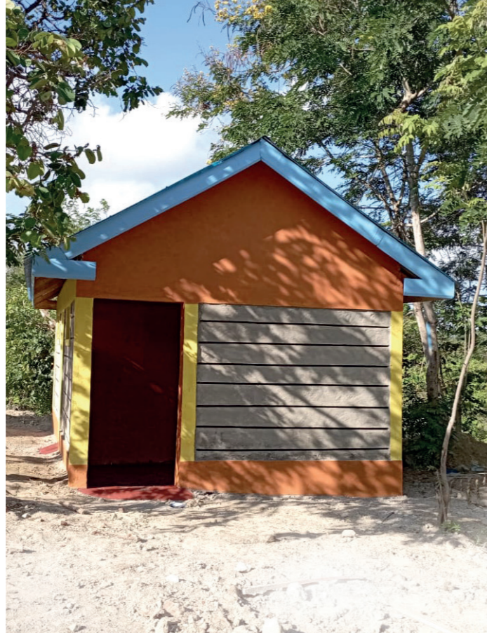
Photo courtesy of Raising Futures: new school toilet block, Kenya
